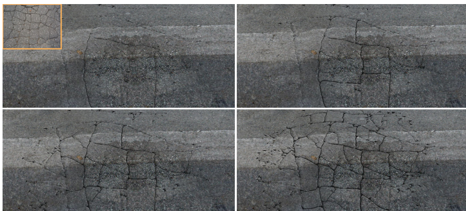
Figure 2.4 – From left to right and top to bottom: road model showing fracture propagation, simulating the course of time with our physically-based aging simulation of brittle fracture [Glondu 12a]. The inset is a photograph of a real road.
