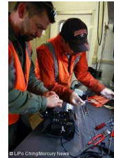
Fig. 1. Crew splicing fiber-optic cables.
