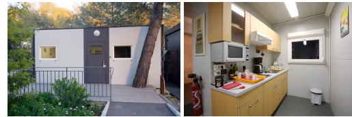
(a) External view of the experimental apartment (b) The kitchen in the experimental apartment
