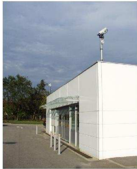
Fig. 9. The two cameras installed on the parking
