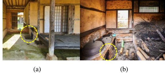
Fig. 3. Ondol Combustion Room Entrance (Kitchen) [14].
