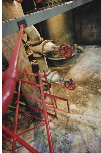
Fig. 4. Head valve of the Lau Balagnas hydroelectric power plant. (©EDF – Gilles de Fayet)
