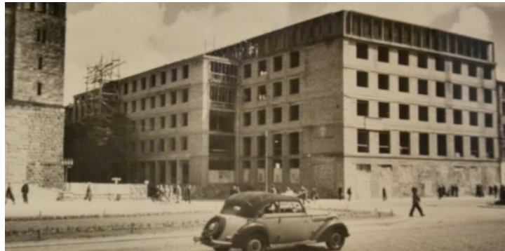
Fig. 14. Construction of the communist party regional committee (around 1950)
