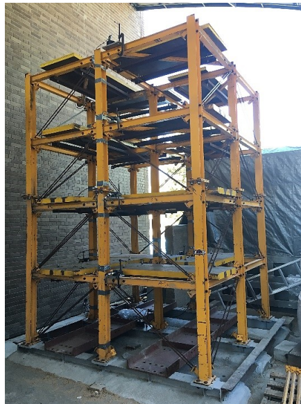
Figure 9: Photo of the Yellow Frame structure (south-east corner).
