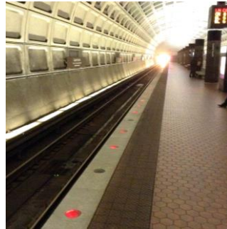
Fig. 1. An LED floor display used in the Washington metro (YouTube ID: DppgBi0ZMc8).
