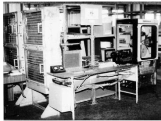
Figure 5.6: The MESz-1 computer constructed by László Kozma, in the museum
