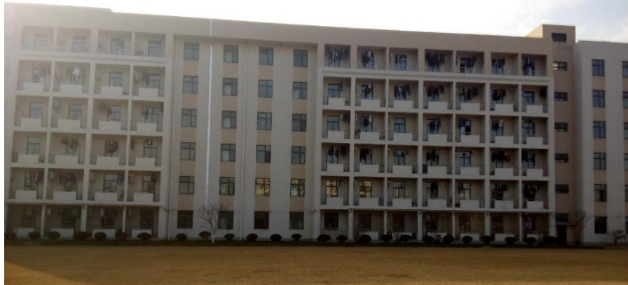
Fig. 4. Facade image of building in campus of Shanghai University.
