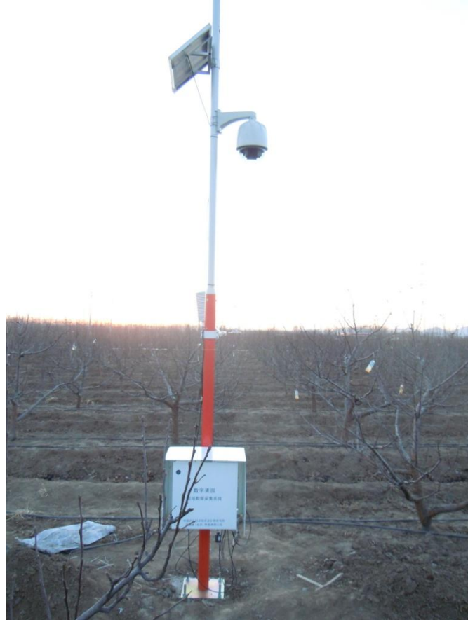
Figure 5. Orchard Field Data Server
