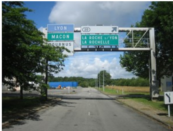
Figure 4: Road sign structure at IFSTTAR
