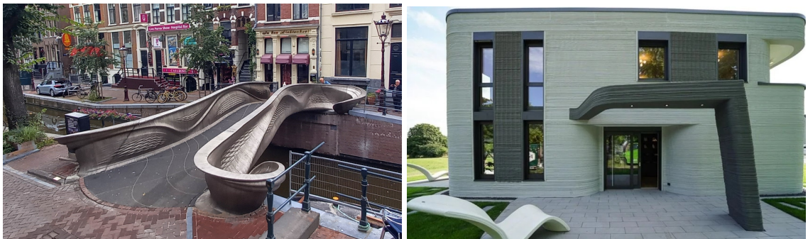
Figure 1: Example of 3D printed objects in cities. Left: 3D printed bridge in Amsterdam designed by Joris Laarman Lab and printed at MX3D. © PersianDutchNetwork, CC BY-SA 4.0 Right: A 3D-printed concrete house © Mense-Korte GbR
