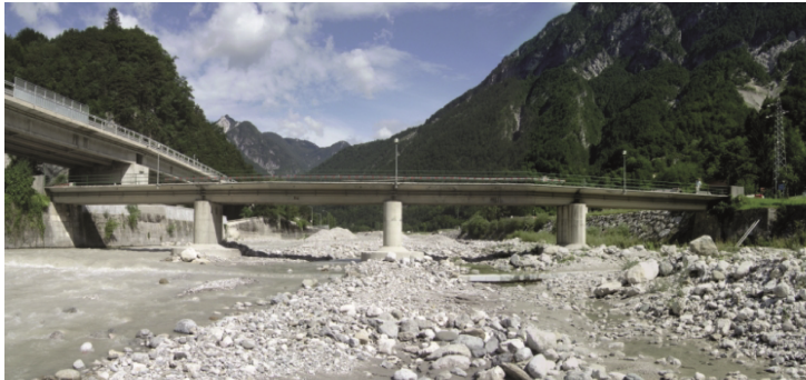
Figure 7.13: Dogna bridge, front view.
