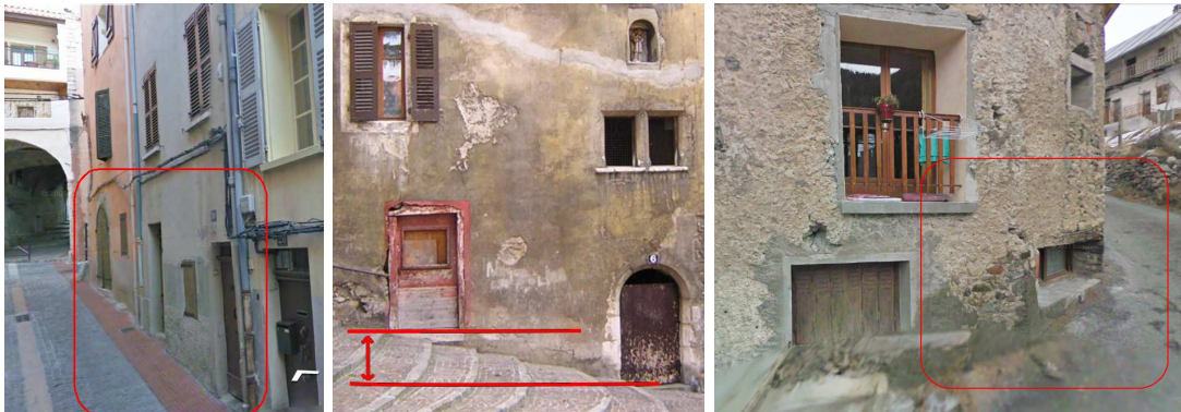
Figure 3.12: Some examples where the architecture of a house has been adapted to the slopes of the underlying terrain.
