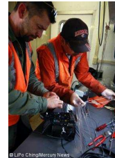
Fig. 1. Crew splicing fiber-optic cables.
