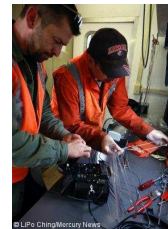
Fig. 1. Crew splicing fiber-optic cables.
