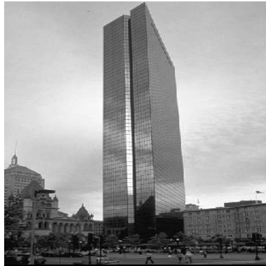
(a) John Hancock Tower, Boston.
