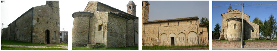
Fig. 9. Canonical views for the pozzoveggiani data set. One image was selected for each side of the church.
