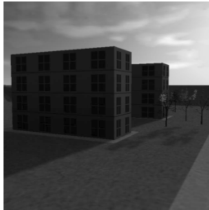
Fig. 7. House from left, view towards the sun.
