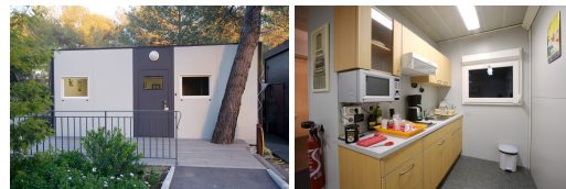
(a) External view of the experimental apartment (b) The kitchen in the experimental apartment
