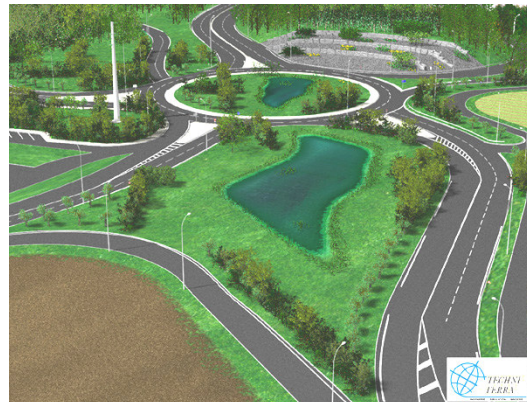
Figure 102 Construction d'un rond-point.
