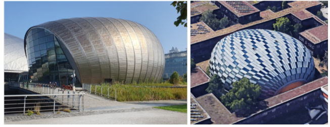
Figure 2: Piecewise developable strips made of glass and steel are characteristic of the architectural style of Norman Foster. Our project aims at facilitating the design of small-scale models for this type of structures. Left: Science Center, Glasgow (photo by the authors). Right: Philological Library at FU Berlin (image from Google Earth: Google GeoBasis-DE/BKG ©2009).
