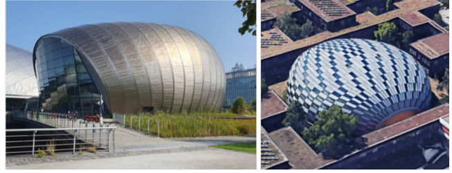
Figure 2: Piecewise developable strips made of glass and steel are characteristic of the architectural style of Norman Foster. Our project aims at facilitating the design of small-scale models for this type of structures. Left: Science Center, Glasgow (photo by the authors). Right: Philological Library at FU Berlin (image from Google Earth: Google GeoBasis-DE/BKG ©2009).
