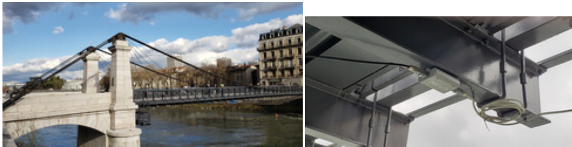
Fig. 1. General view and a measurement node of the Saint-Laurent footbridge.
