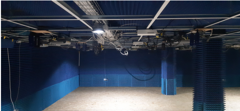
Figure 1: The EM-shielded lab used for the experimental setup.
