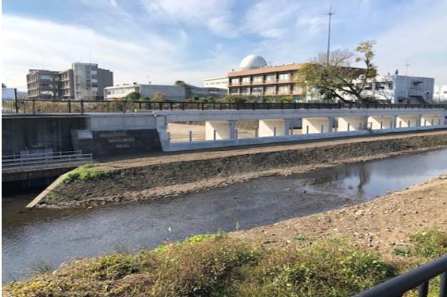
Fig. 10 Rainwater Shelter Storage Pond under expanding construction
