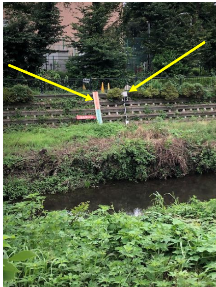
Fig. 9 Nogawa under level 3 alarm
