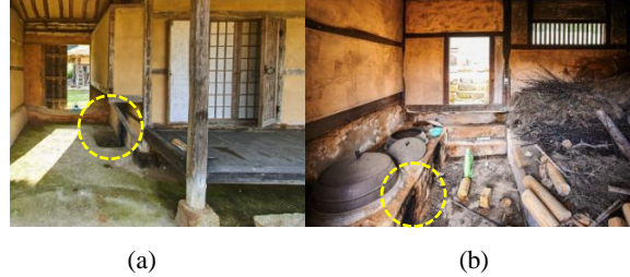
Fig. 3. Ondol Combustion Room Entrance (Kitchen) [14].
