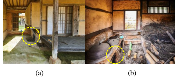
Fig. 3. Ondol Combustion Room Entrance (Kitchen) [14].
