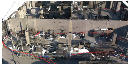
(e) Close-up view of the construction site from GT_3
