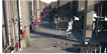
(b) Corridor view of the construction site from GT_1
