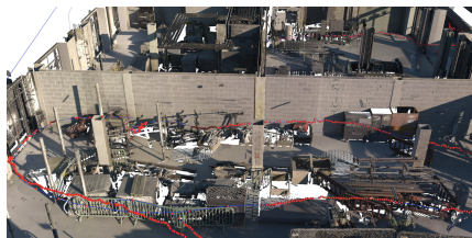
(i) Close-up view of the construction site from GT_5
