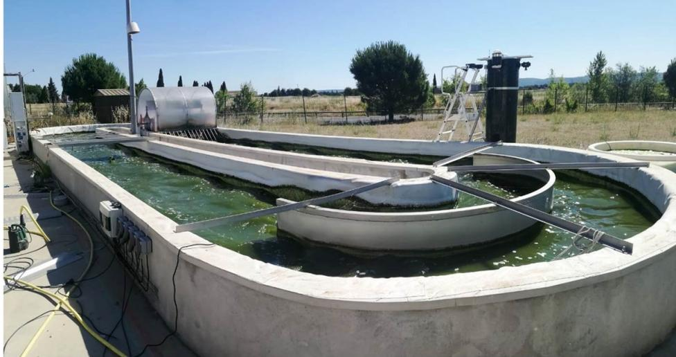
Figure 1: High Rate Algae-Bacteria pond (HRABP) located in Narbonne (F).
