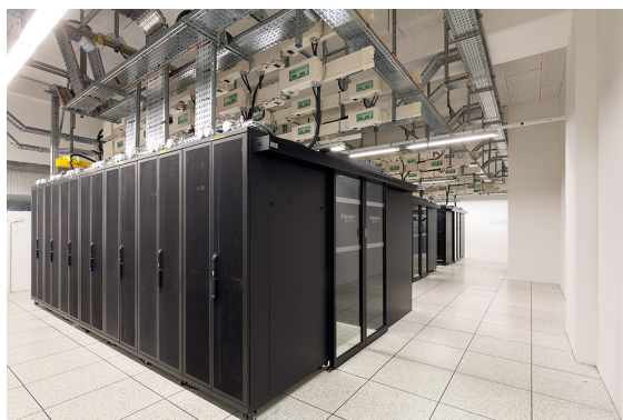
Figure 2.1. General view of the CIMENT cluster at UGA
