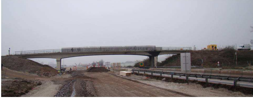
Figure 8: S101 Bridge before demolition.
