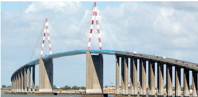
Figure 1. St. Nazaire Bridge, Nantes.
