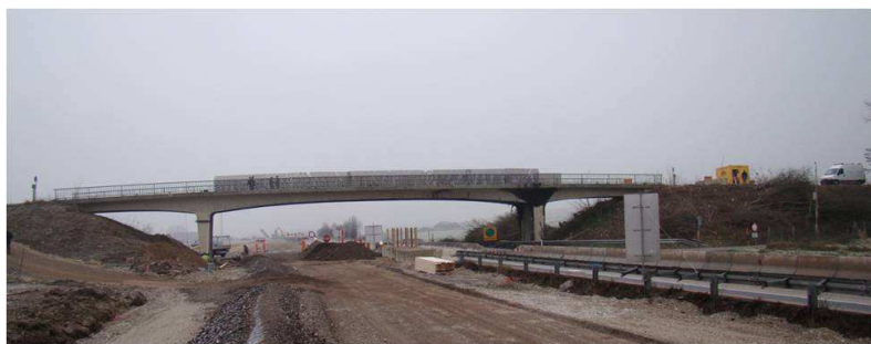
Figure 11: S101 Bridge before demolition.
