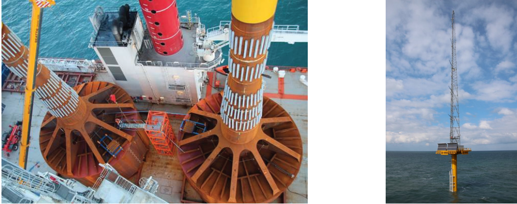
Figure 7: Twin Mono Bucket foundations on board of the installation vessel (left). Meteorological mast at Dogger Bank (right). Both photos available by the courtesy of Universal Foundation A/S.
