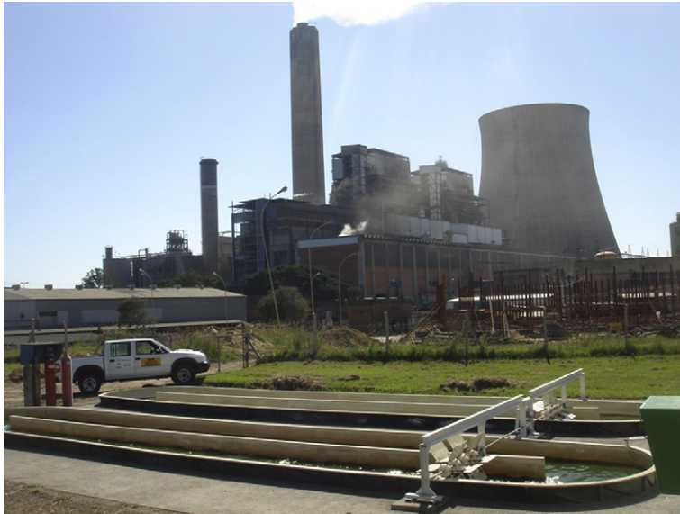
FIGURE 1.2 Cultivation of Spirulina for the CO 2 biofixation that is emitted in the combustion of coal in a thermoelectric power plant (UTPM, Brazil).
