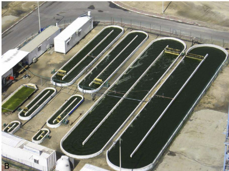
FIGURE 2.8 (a) Sapphire's green crude farm with raceway open ponds ( www.sapphireenergy.com/rendition.medium/images/multimedia/green%20crude%20farm%20ponds.jpg ). (b) Seambiotic's pilot plant ( www.seambiotic.com/uploads/Seambiotic%20Ltd.%20-%20Algae%20Pilot%20Plant%20white%20paper.pdf ).
