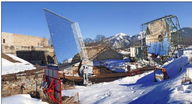
Fig. 4. Solar furnace with double reflexion in Mont-Louis, France.
