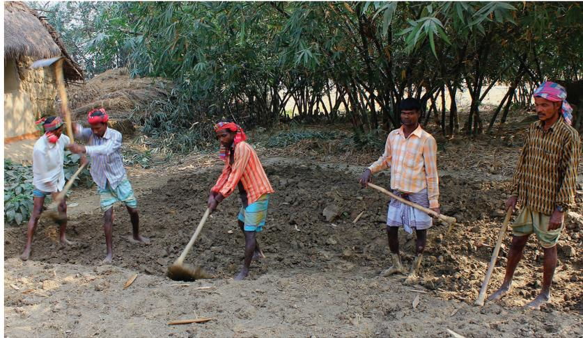
Extraction and preparation of earth for construction
