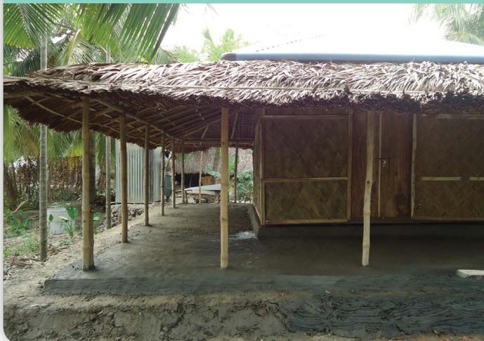
**Materials:** mud, bamboo, reinforced concrete posts, corrugated galvanised iron sheets, tiles, golpata, wood
