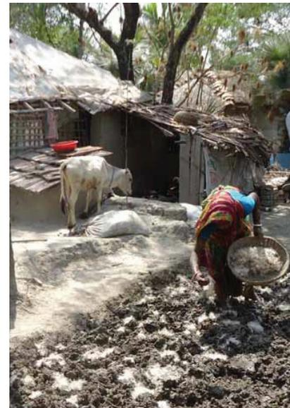
Earth and fibre for cob walls production
