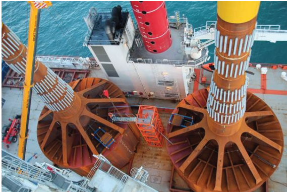
Figure 1: The Mono Bucket foundations for the masts at the DB.
