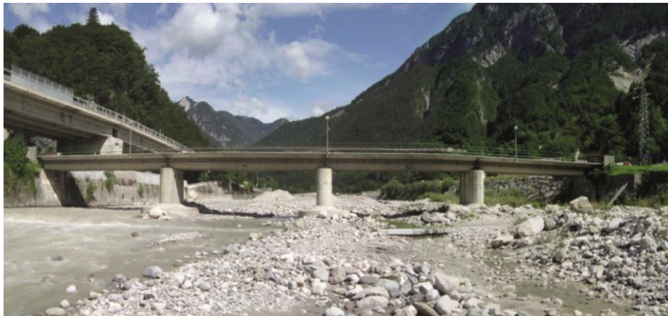
Figure 2. Dogna bridge, Italy, after [17].
