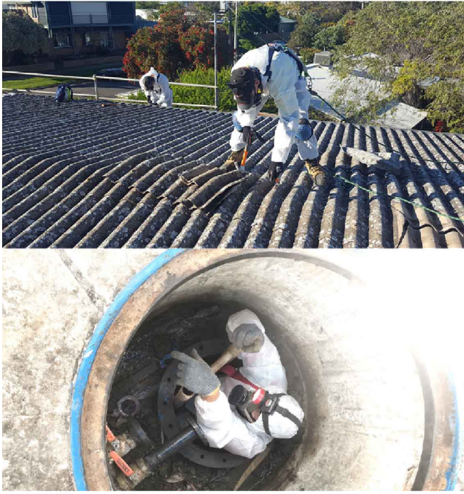
Fig. 2: Examples of hazardous working environments where robotic avatars could replace humans. Top: Asbestos tiles removal operation. Bottom: Maintenance operation in a confined space for oil and gas.
