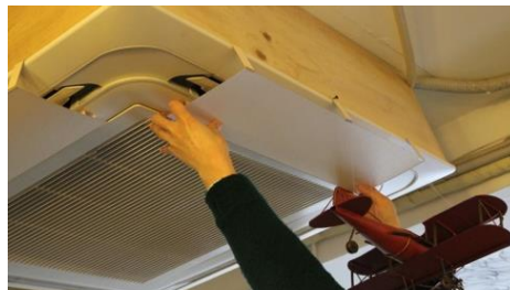
Fig. 8 Wind guide plate to divert cold wind from air conditioner to other direction
