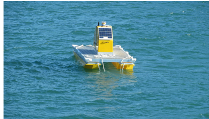
Fig. 2. Avoid hard-accessible places, if possible. To achieve this platform, the technicians needed about 45-minute boat drive. They installed the platform (incl. motes and a GSM modem) but had to come back here after a few days only to update software.
