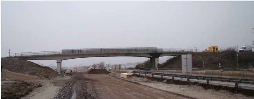
Fig. 6 Bridge S101 during damage test [23].
