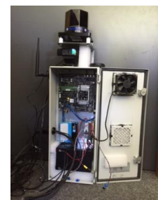
Connected Perception Unit
