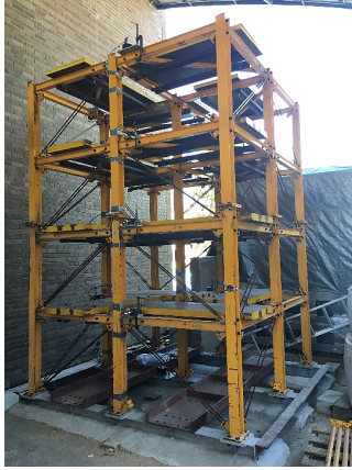
(a) Photo of the Yellow Frame structure (south-east corner)
