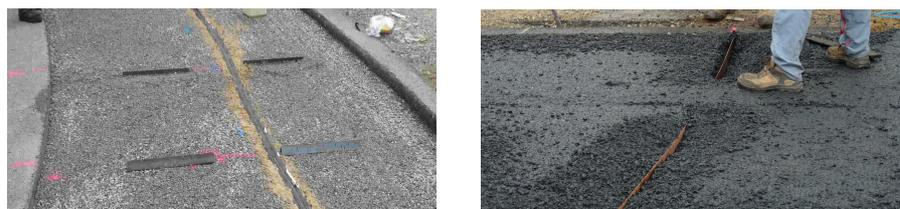
**Fig. 2** Photographs showing the different types of steel bars embedded in the asphalt.
