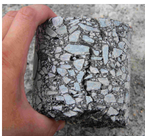
Fig. 13 Photograph of the cores taken from the DGBM structure.
