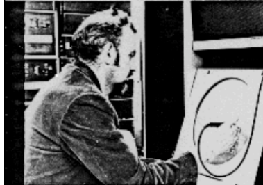
Fig. 1: The MINNIE interactive-graphic CAD system, 1968
